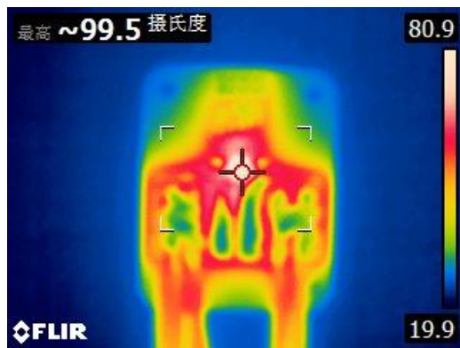
Package Thermography (Input Current 40A)
